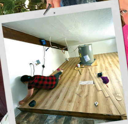
Dawn laying flooring at the ministry house. May, 2024.
